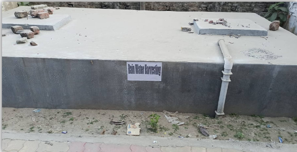
Fig. 3 Rain Water Harvesting UG Tank
